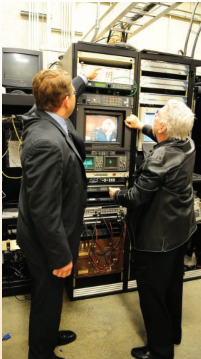
Paul looked over the station's transmitter equipment with Ron Kasper, WSEJ vice president of operations and engineering.
