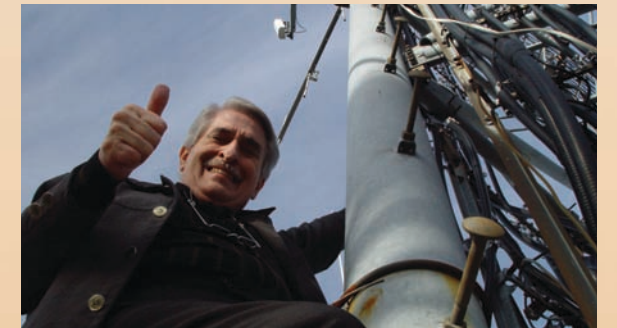
Paul at TBN's new digital TV transmitter tower covering New York City!
