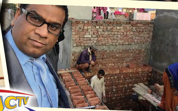
Pastor Javed Rauf of JCTV-Pakistan at the construction site of the new TV studio in Lahore, Pakistan.
